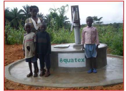
Completed Community Hand Dug Well at Hangha, in the Kenema District, Sierra Leone
